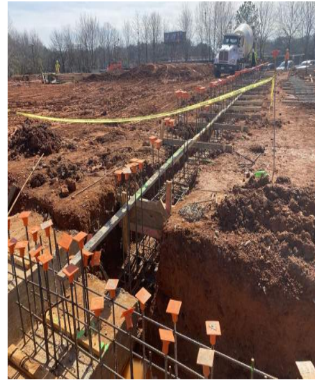
Footing prep for inside block, parallel to grid line D, 20' north
