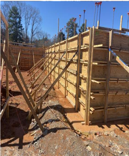
Continuing formwork for foundation walls
