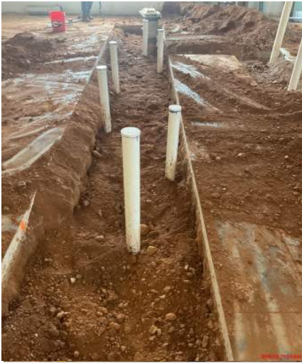
Rough-in plumbing at serving line area
